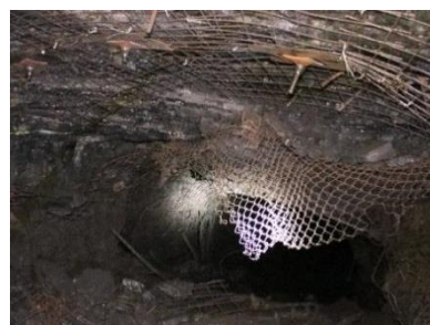
Figure 1. Deformation of upper layer transport roadway.
